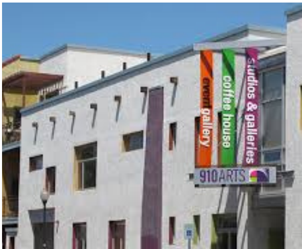
Front of Building
